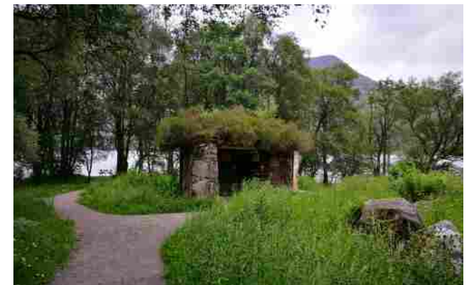
Figure 68: Example of green roof at tourist information shelter
