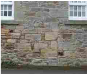
Sandstone rubble wall
