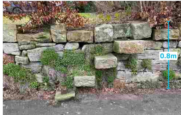
Figure 53: Mounting steps with squared crenellation coping, Eglington
