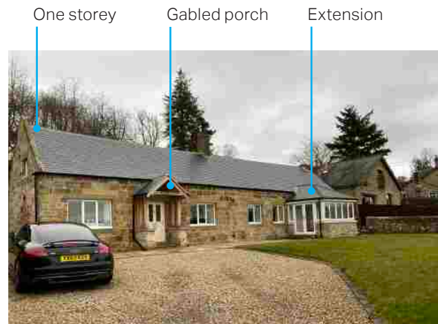
Figure 66: One storey conversion in Eglingham
