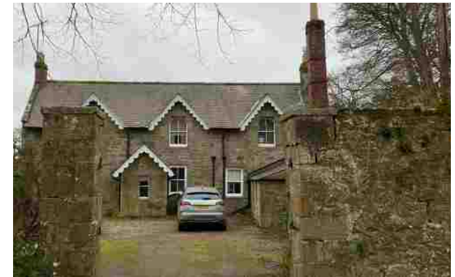
Figure 43: 2-storey detached property in Eglington
