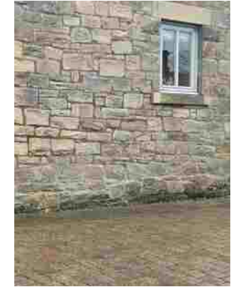
Figure 73: Natural stone (sandstone) is used as the main building material and brick used for some surfacing
