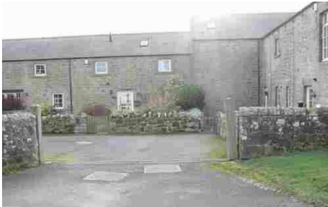
Figure 47: Farmstead conversion in North Charlton
