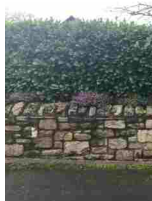
Figure 74: Boundary walls are similar to the local stone wall field boundaries
