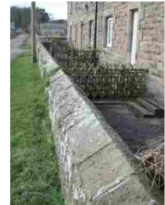
Figure 55: Saddle (pointed) coping stones, North Charlton
