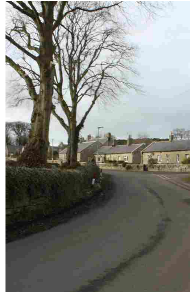
Figure 1: South Charlton streetscape
