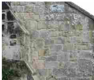
Loosely laid courses
