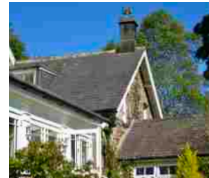
Split level roofs
